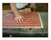
2. Cut the panel at a 45 degree angle. TIP: A simple panel cutting jig helps to do this on a table saw.
