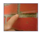
For a final finish, use Texture Plus<sup>®</sup> color-matched caulk to fill all screw holes and any gaps.
