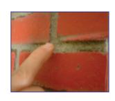
For a final finish, use Texture Plus° color-matched caulk to fill all screw holes and any gaps.
