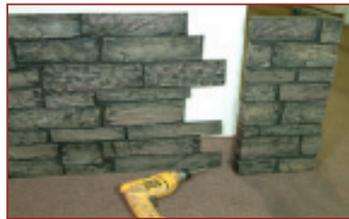
2. Next, overlay the molded corner directly on top of the panel.
