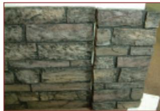
2. Align a Texture Plus® **standard** panel (or trim an **interlock** panel) to the molded corner.
