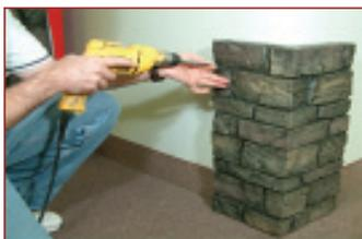
1. First, attach molded Texture Plus® corner to wall by applying glue to the backside of the corner and screwing into wall.
