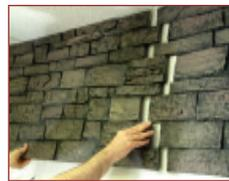
8. Fit the next panel and glue and screw in place. Repeat until the row is complete.
