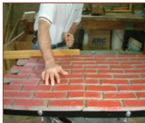
3. Take the leftover panel and flip it around 180 degrees. You will be cutting a 45 degree angle reversed to the last cut.
