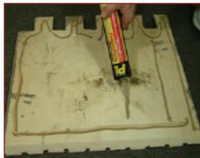
5. Then take the first piece and apply glue to the back of the panel.
