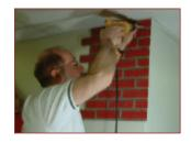
6. Fit the glued piece. Screw it to the wall.
