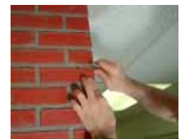
roll edges with a rounded object
