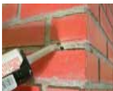
fill screw holes/gaps
